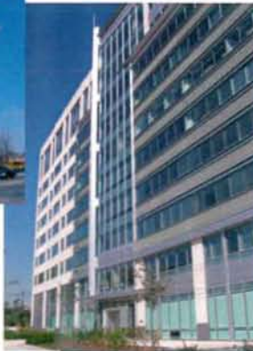
1100 New Jersey Ave, SE Federal Gateway Building New Jersey Ave (West) Facade
